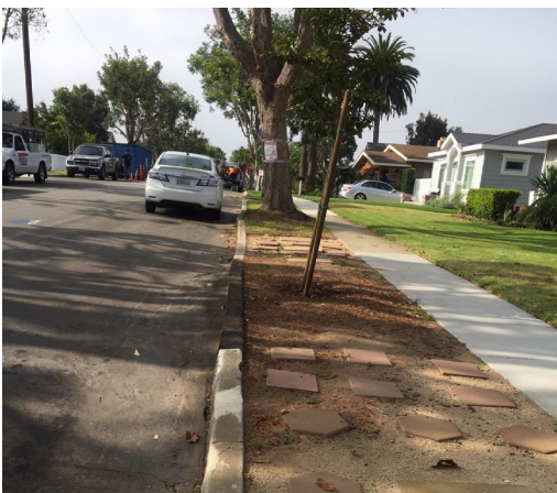
Before: 423 Whiting St. asphalt curb in front of the new tree, non-straight curb
