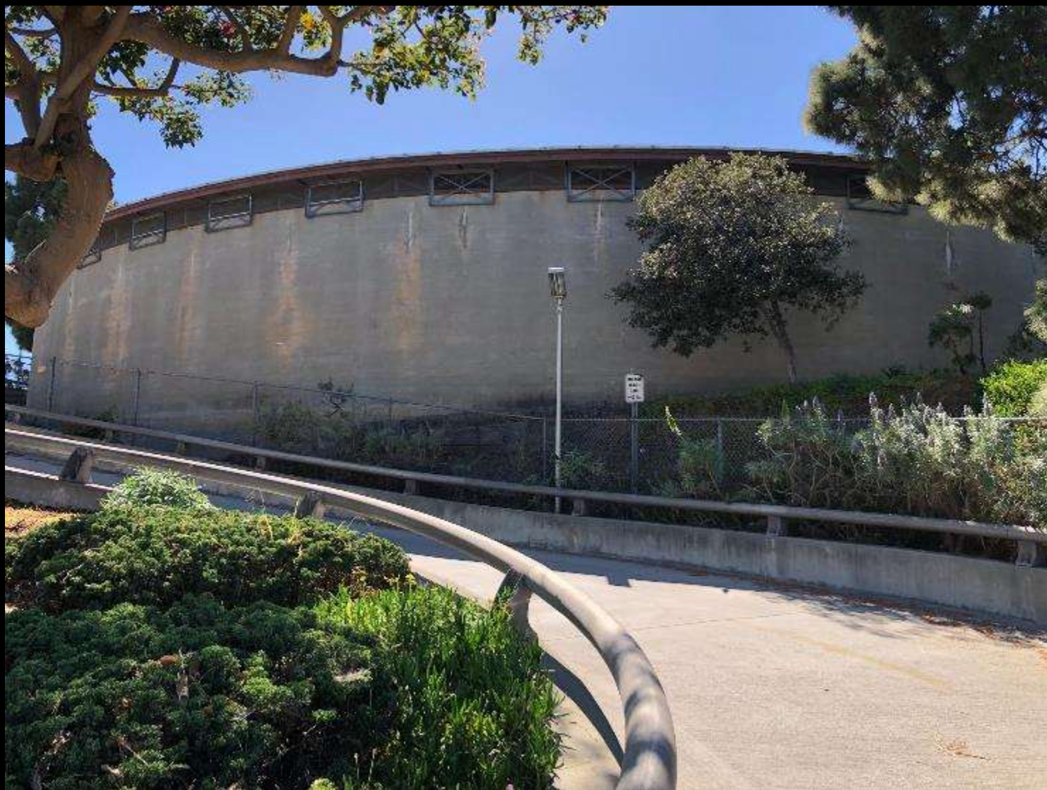
Potential wall for mural at the Water Operations off Maryland Street (wall facing east).
