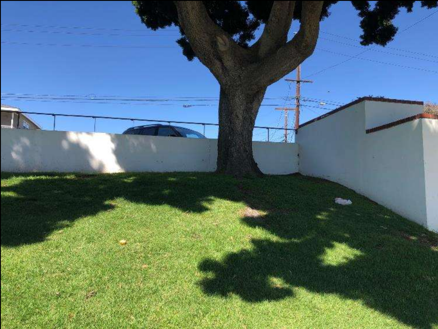
Potential walls for murals left of the George E. Gordon Clubhouse (walls facing south).
