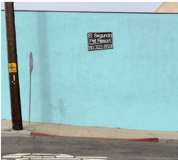
Before: 231 E. Franklin, unused driveway approach on Eucalyptus side
